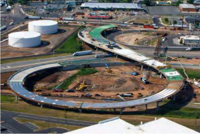
One of the many big jobs completed by D'Annunzio & Sons.
